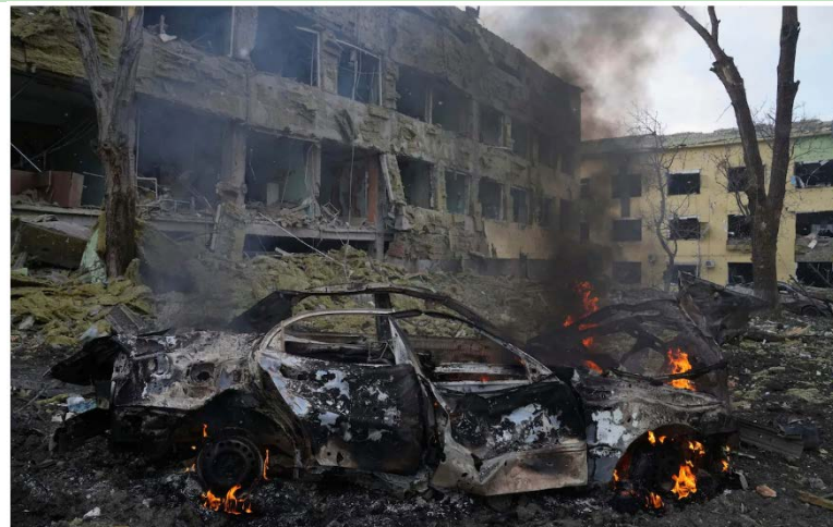
A car burns outside a maternity hospital damaged by shelling in Mariupol | CREDIT: AP Photo/Evgeniy Maloletka
