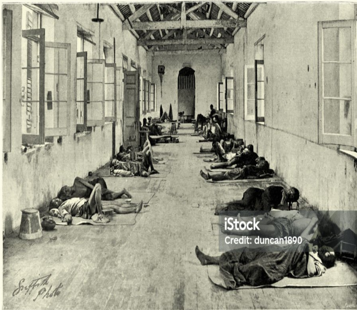
"In this time of need for the accommodation of the sick these glass works have been converted into a temporary hospital, and are now a receptacle for the worst cases. The two large rooms forming their wings are the separate wards for the men and women. The sick have mat beds, where, left in their dirty clothes, they may die or struggle through the disease"
